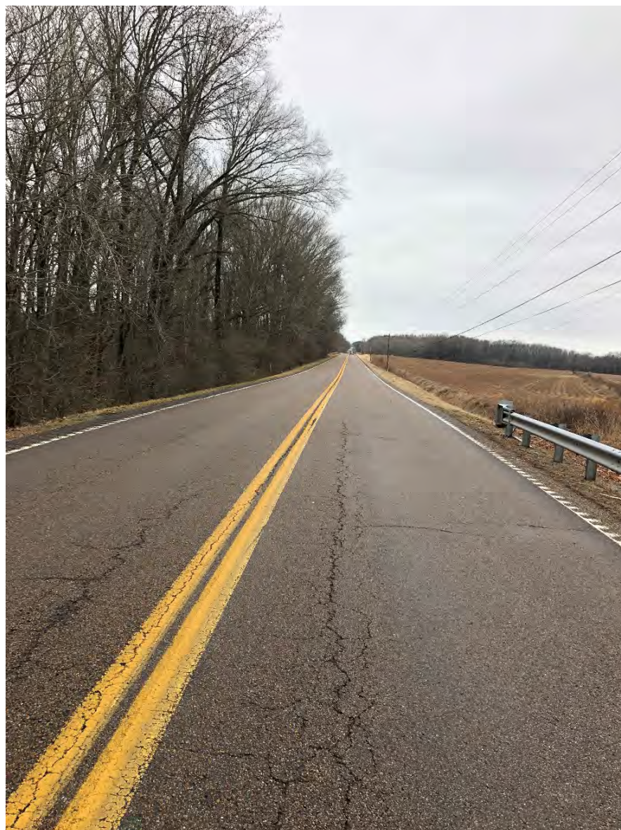
Looking West from Bridge
