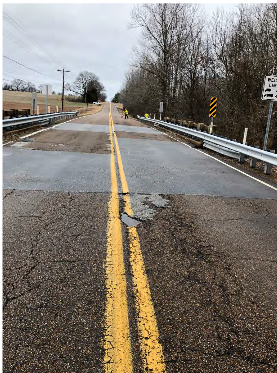
Eastbound Approach to Bridge
