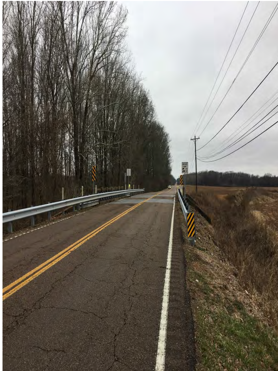
Westbound Approach to Bridge
