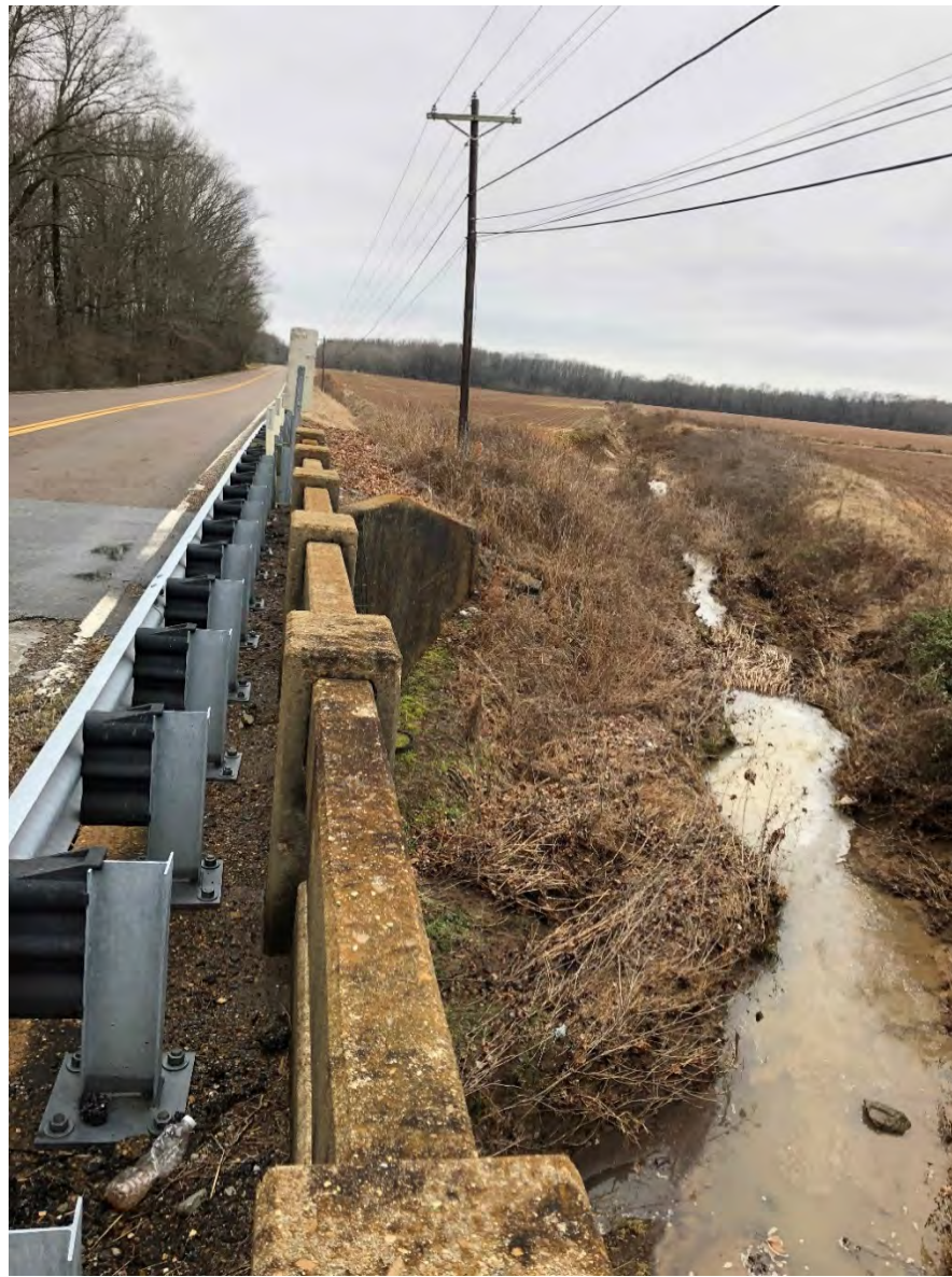
Utility Poles on North side (Downstream) of Bridge
