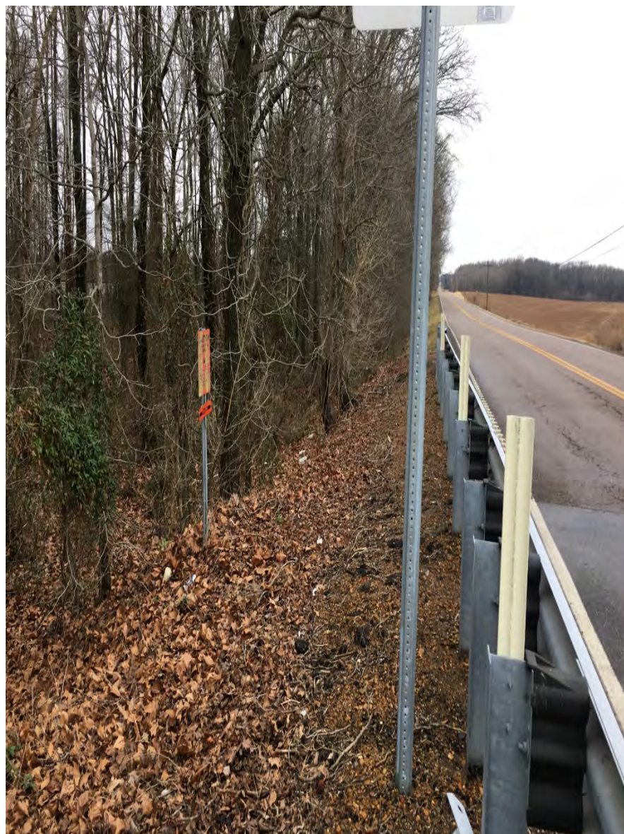
Fiber Optic Cable Utility Sign, Southwest of Bridge
